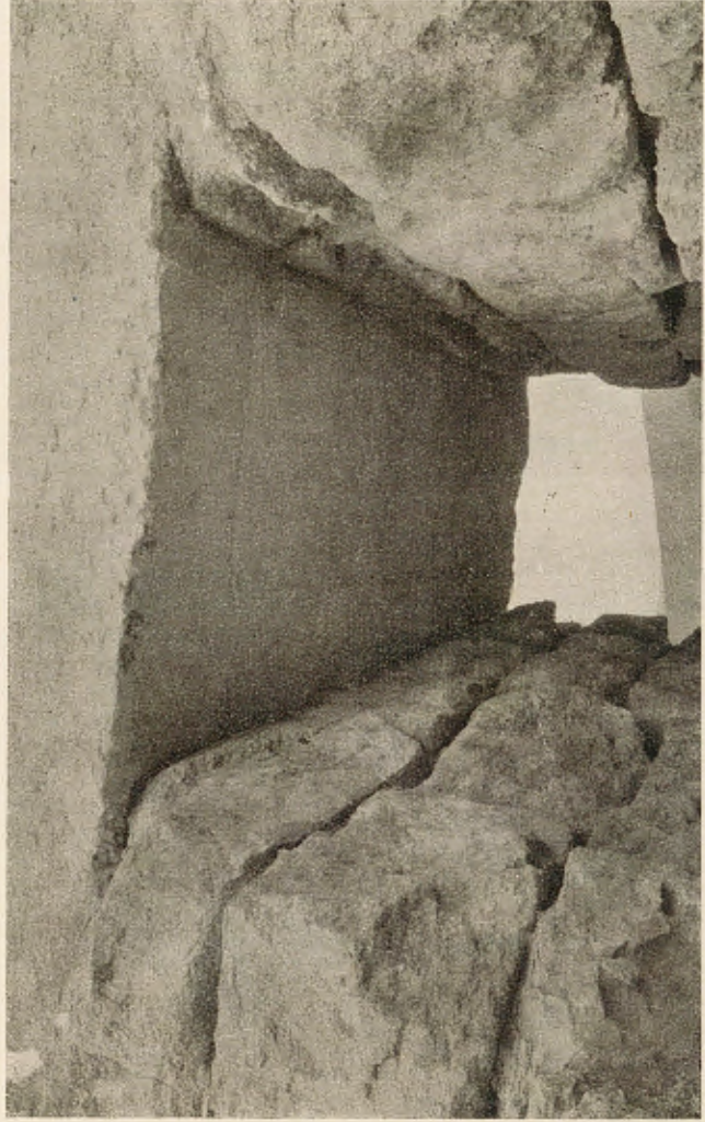
View showing underside of the slabs.
